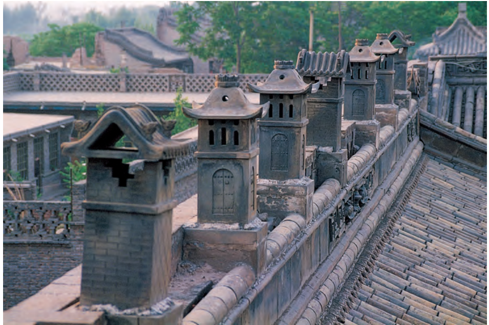
The Qiaos' House abounds in decoration. The picture shows the chimneys on top of the roof, which are well decorated despite the
