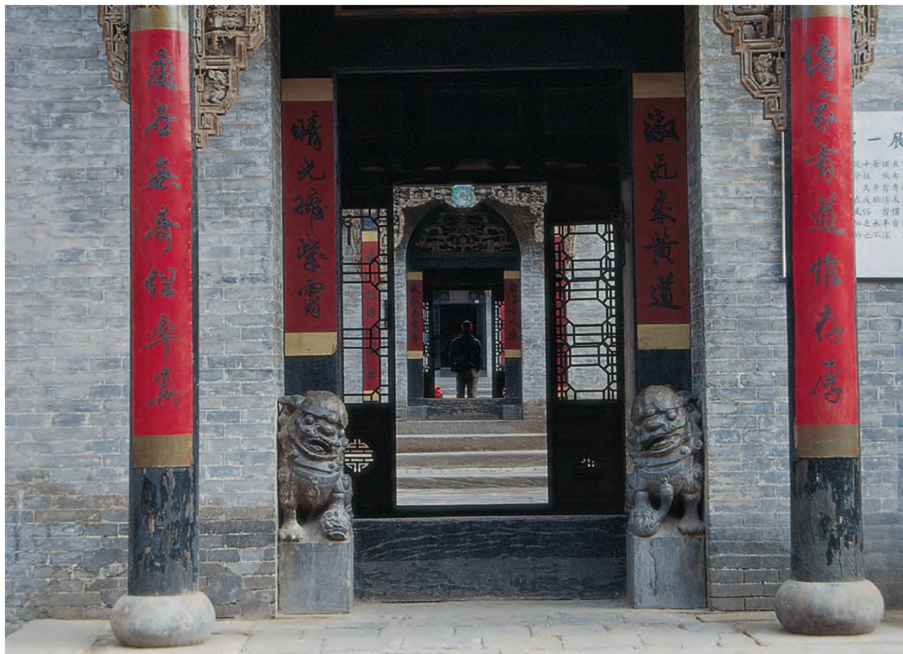
The Qiaos' House, a representative of the traditional rural residences of Qixian, is a museum of folk culture today. The picture shows the entrance to
